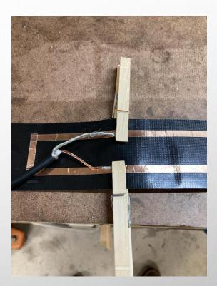
Step 5: Permanently\* attach feedline tail to antenna with small screws or pop rivets
