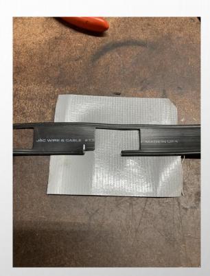
Step 4: Expose ladder line wire between 2-1/2" and 3-1/2" up from the bottom
